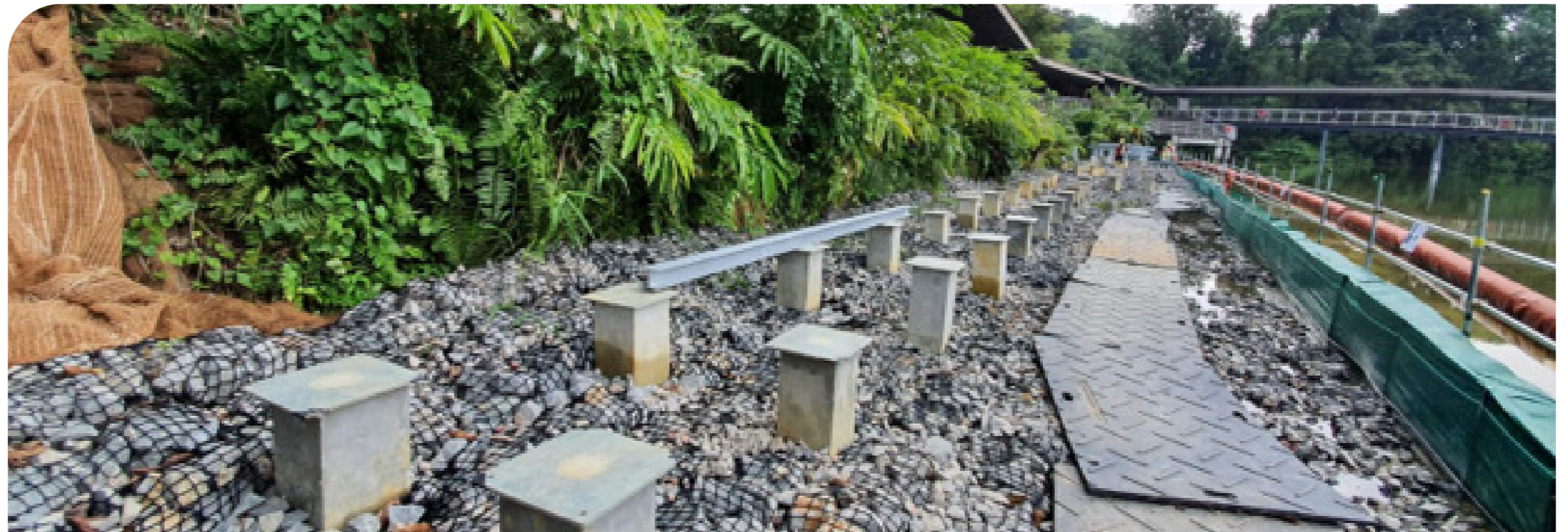
RIGHT: Phase 1 works with shoreline protection for the Boardwalk.
