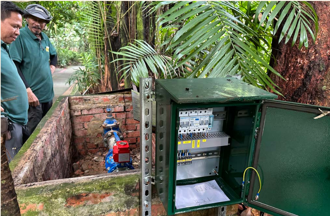
Facilities Management team inspecting the meter and motorised valve installed at one of the potable water branch lines.
