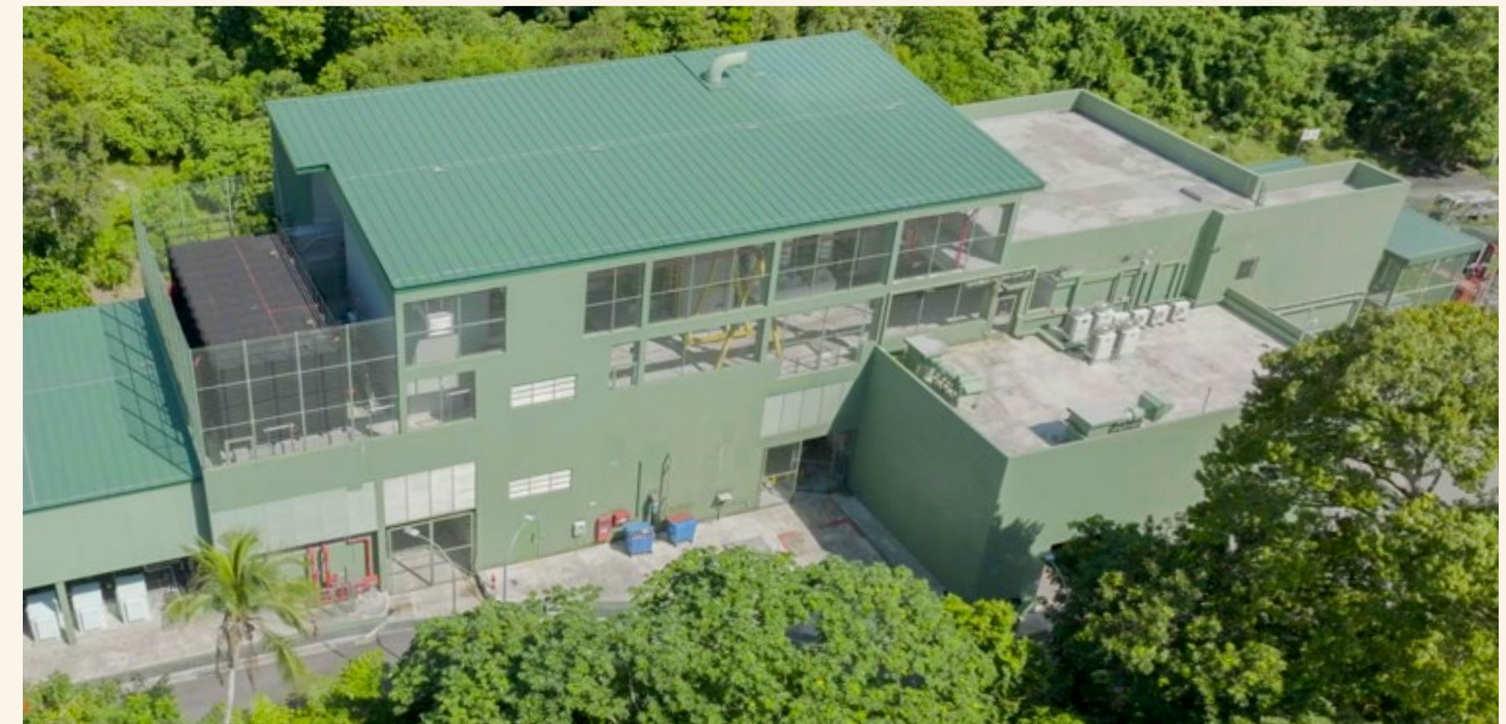
An aerial view of our wastewater recycling plant.
