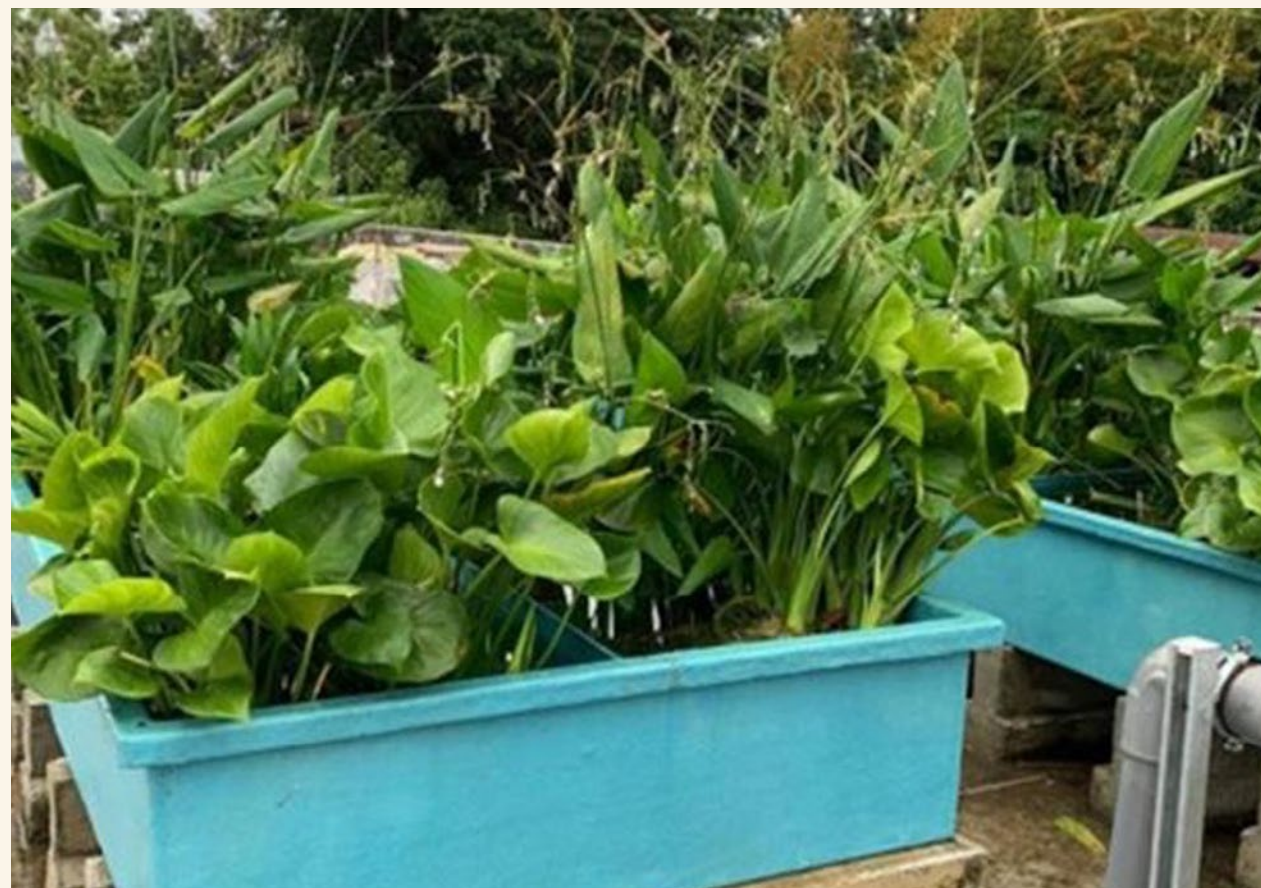
The bio bed filter system at River Wonders recycles wastewater using plants like pandan and alligator-flag.
