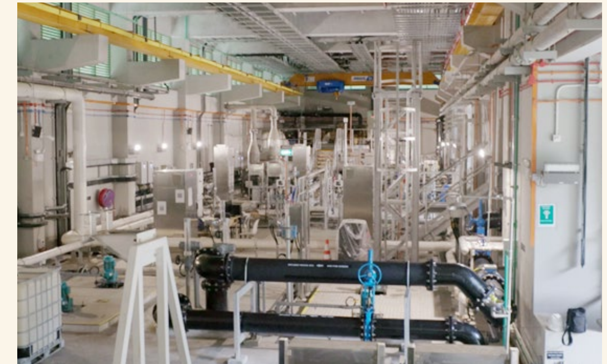
The advanced wastewater recycling plant transforms animal wastewater into high-quality, non-potable water for park use.
